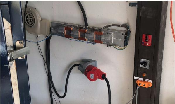
Now the pi controller manages this one power brick, but with the 3-phase wall jack I mounted to its output I could select which oven I plug in at any time.
